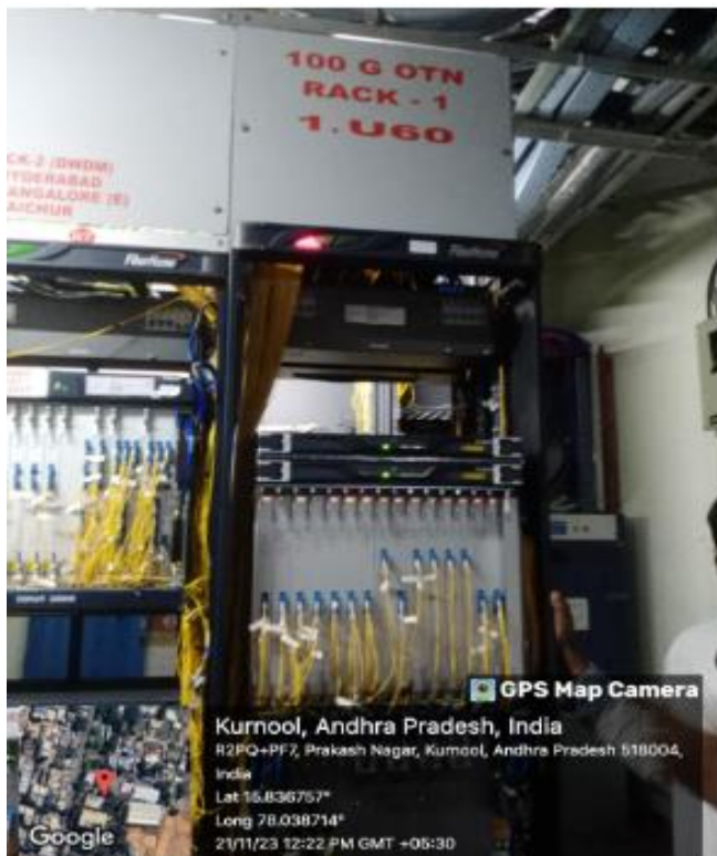
Fig: Ethernet photo
